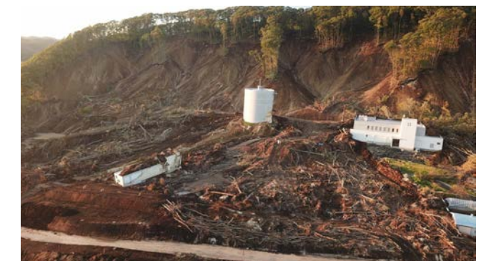
Drone image of landslide damage to a critical water treatment plant during the 2018 Hokkaido Earthquake. Photo courtesy of GEER
